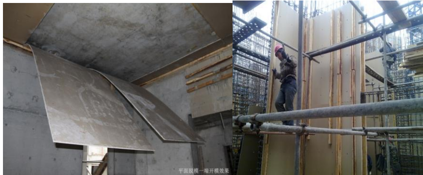
Wood + Plastic shuttering ply-like board making
